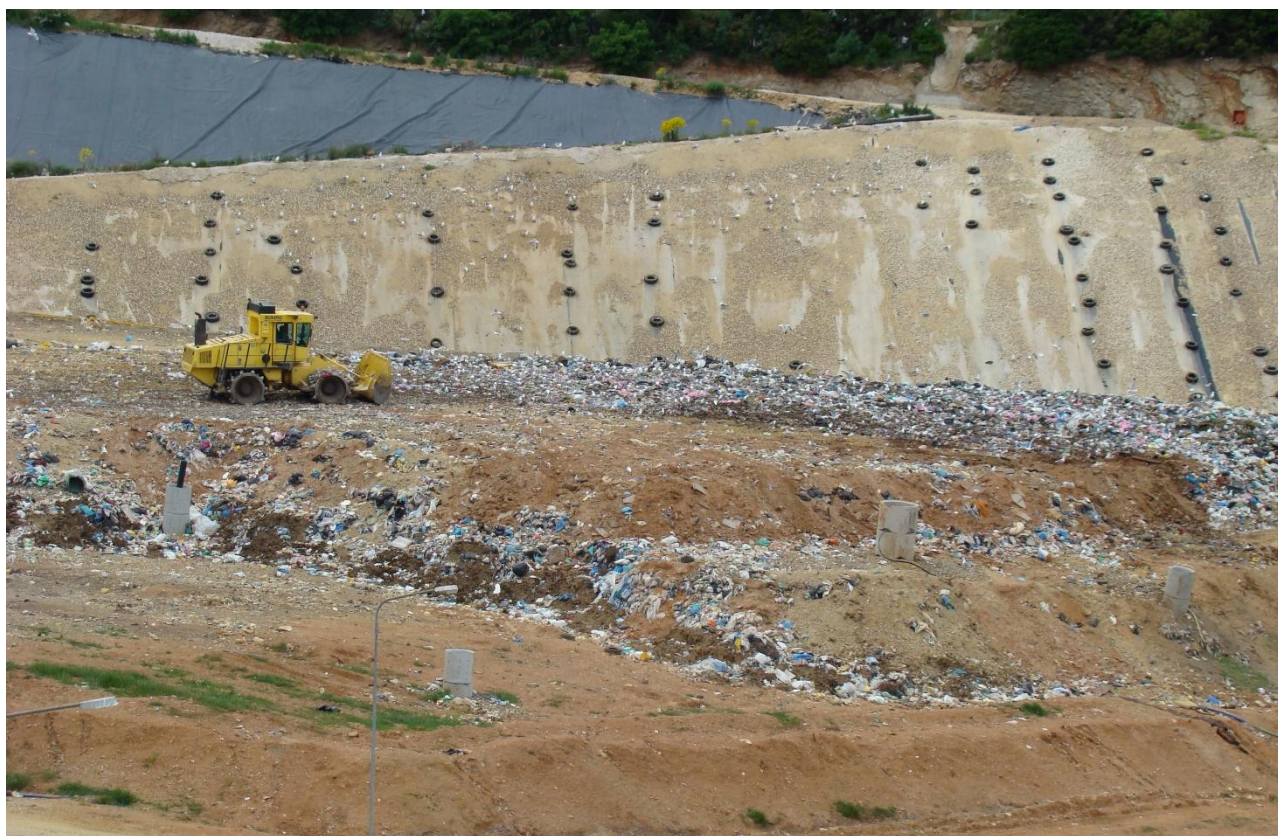
Photo A2. Details of the disposal and compacting operations at the current disposal cell
