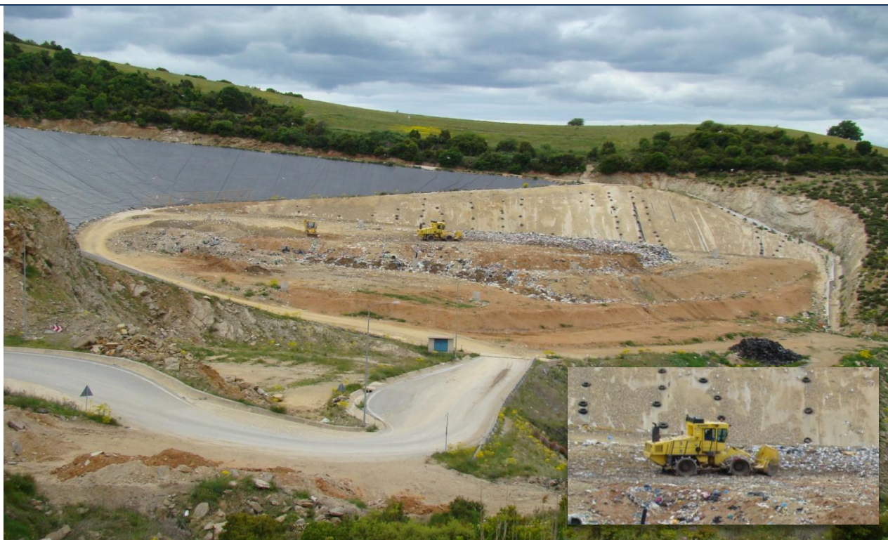
Figure 9: View of the PL disposal area and details about the layering and compaction operations taking place at the current working cell
