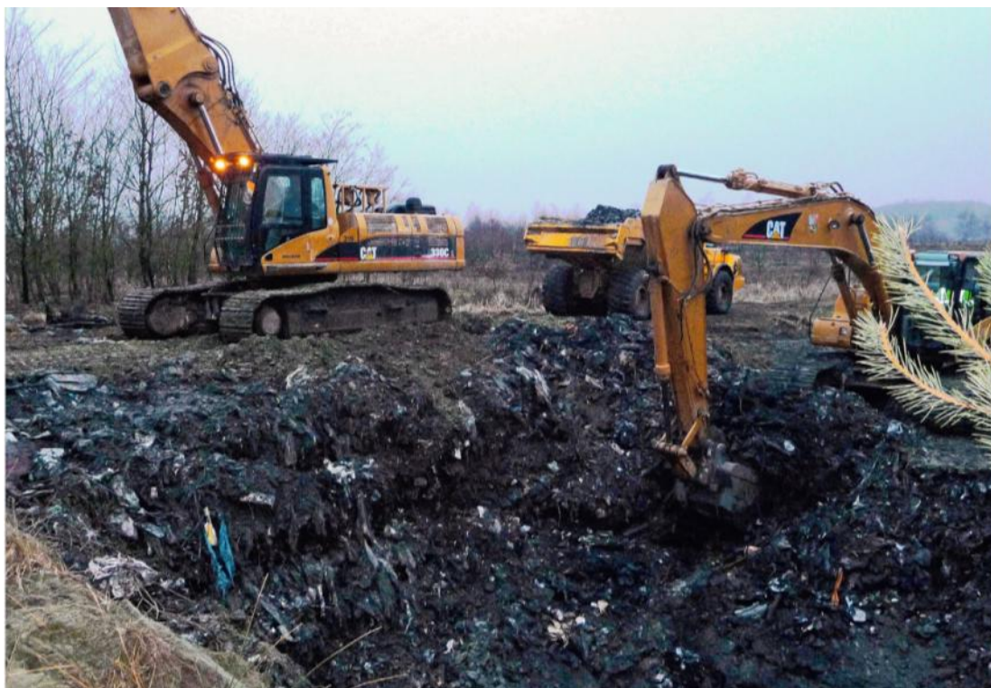
Figure 13: Typical application of top excavation in landfill mining operations using excavators and dump trucks
