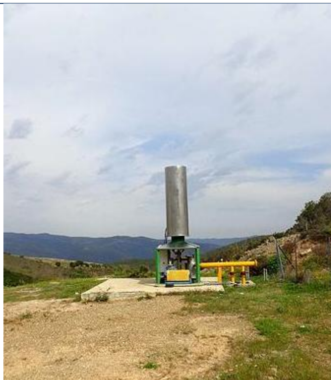
Figure 4.3.1-6: Torch for burning the biogas from the landfill cell, Polygyros Landfill
