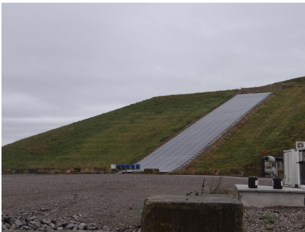
Figure 4.2.2-4: Solar panels, soft use for an old landfill (Antwerp landfill, Belgium)
