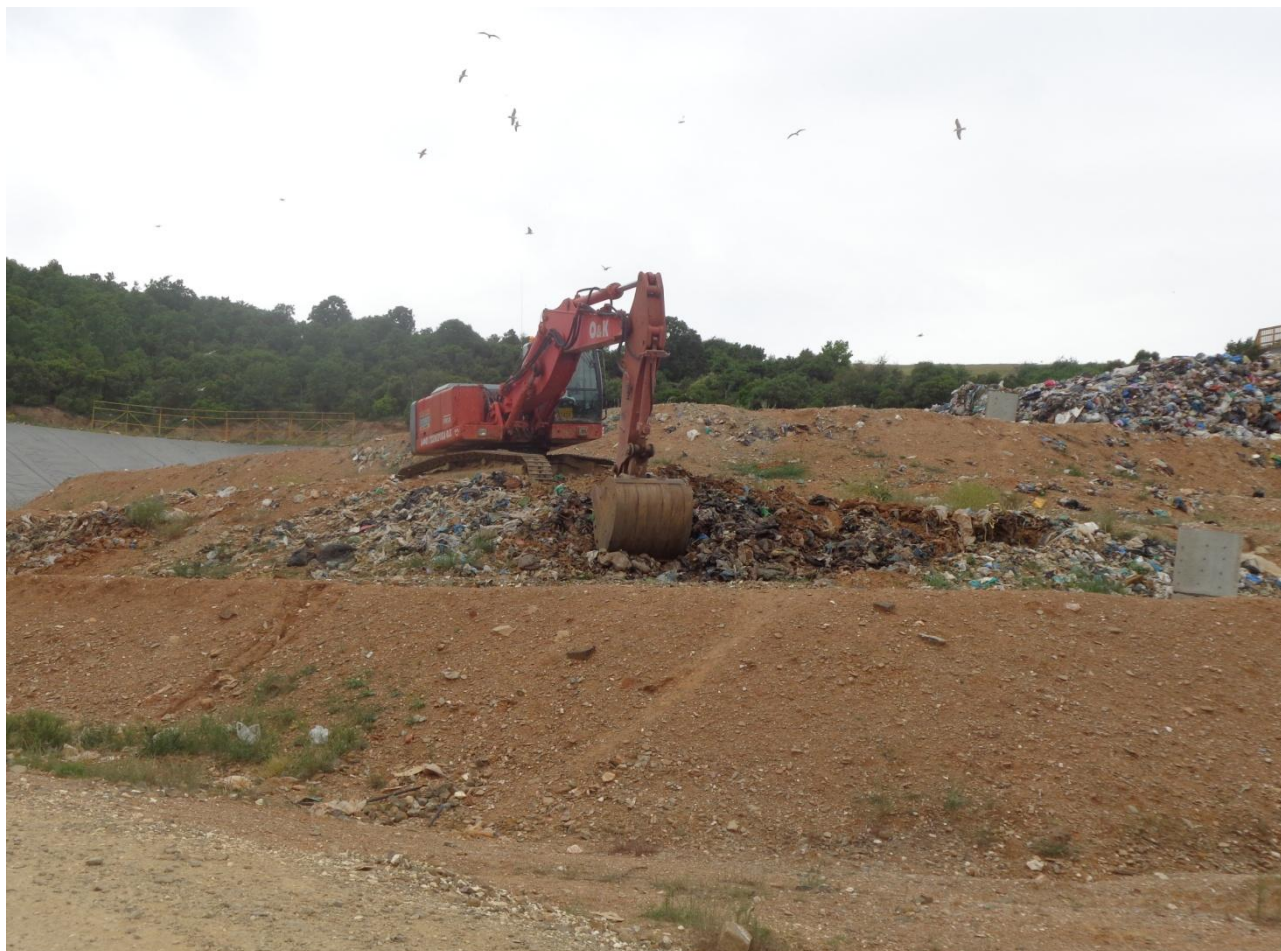
Figure 3.1-4: Application of the top excavation method in the landfill mining area
