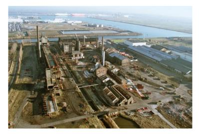
Closure and remediation of a former steel cokes manufacturing plant. Full demolition. No conservation due to high pollution (PAHs, heavy metal,...).
